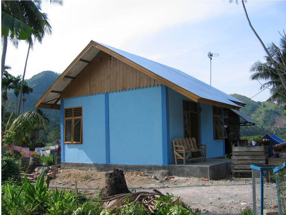
*Confined masonry is the most commonly preferred structural system by homeowners in Aceh, Indonesia, shown here. In partnership with a team of pro bono structural engineers, Build Change performed engineering analysis and developed confined masonry structural design drawings for this typical single family house.*
