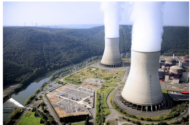
Figure 3: Example of a power plant with cooling towers that could potentially benefit from the Infinite Cooling technology
