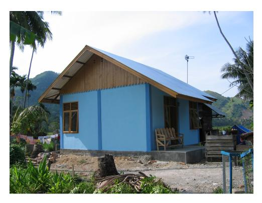
Confined masonry is the most commonly preferred structural system by homeowners in Aceh, Indonesia, shown here. In partnership with a team of pro bono structural engineers, Build Change performed engineering analysis and developed confined masonry structural design drawings for this typical single family house.
